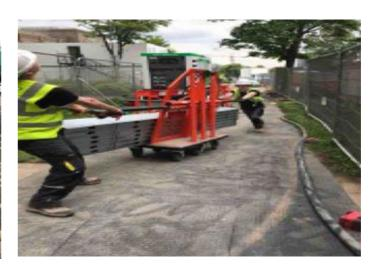
The trolleys are also fitted with a deadman's, brake where both brake levers must be depressed in order to move the unit. This ensures that movement of the trolley is a safe, two-man operation.
