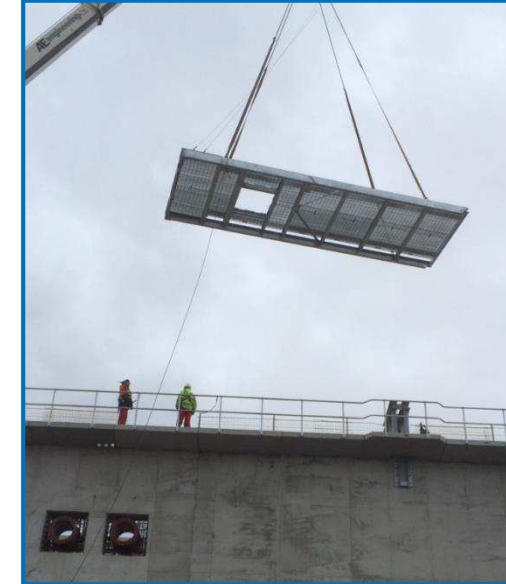
Lifting with Eye Bolts
