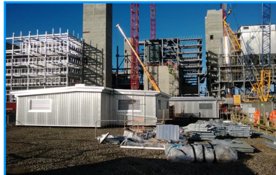
Erected Half Module - Top Right
