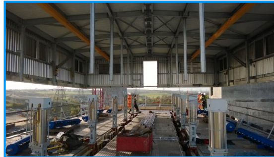
Module Being Lowered.
