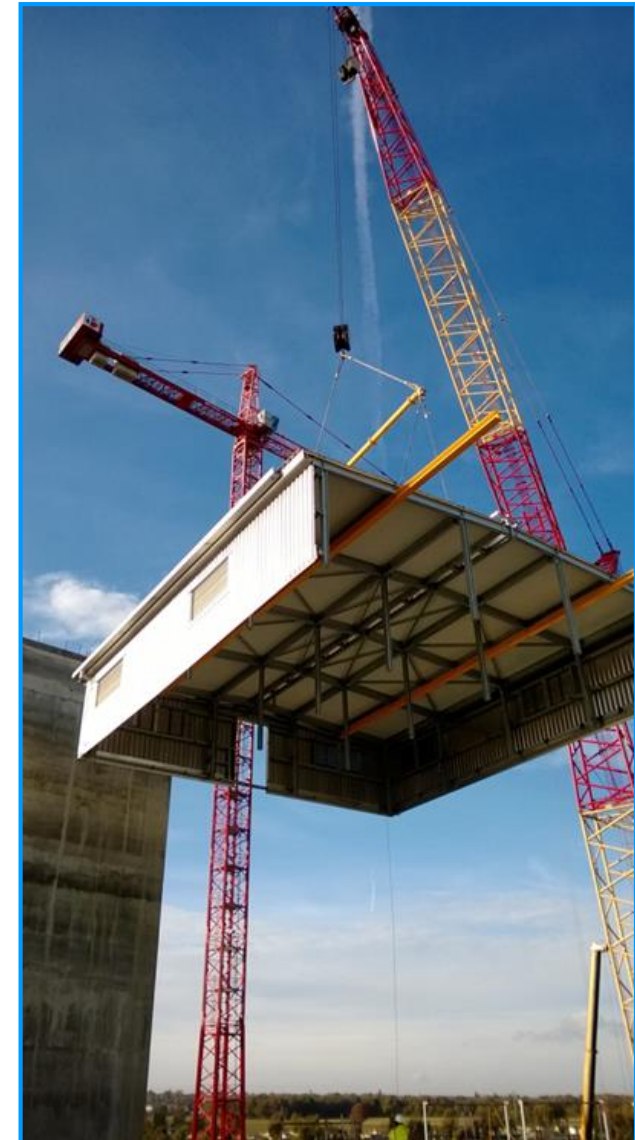
Module Being Lifted
