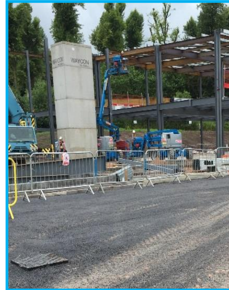
Installed Shaft Units
