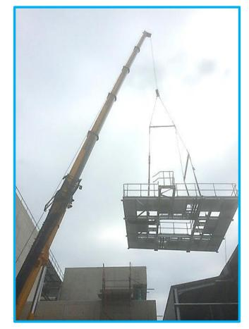
8 N° high level Decanter floors were split into 14 N° units per floor and built up offsite. The units were stacked 5 high with timber spacers. The units were stacked in the erection sequence order to save time onsite (Left).
