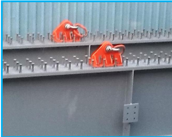
Lifting Lugs on Beams
