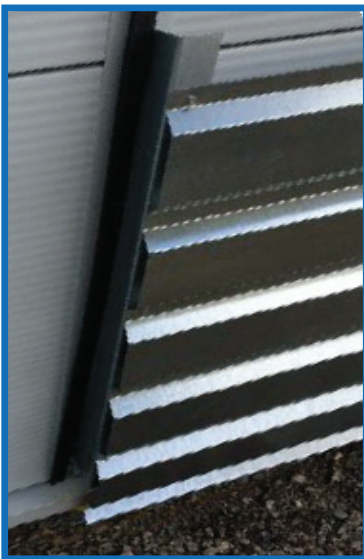
Rail End Fixing
