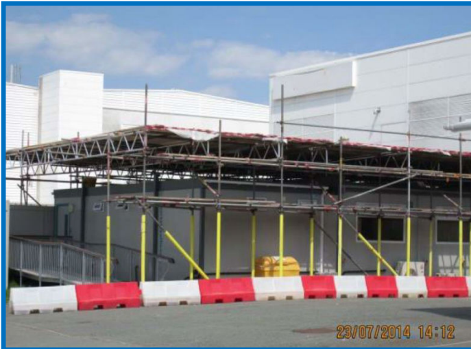
Design Scaffold Over the Office
