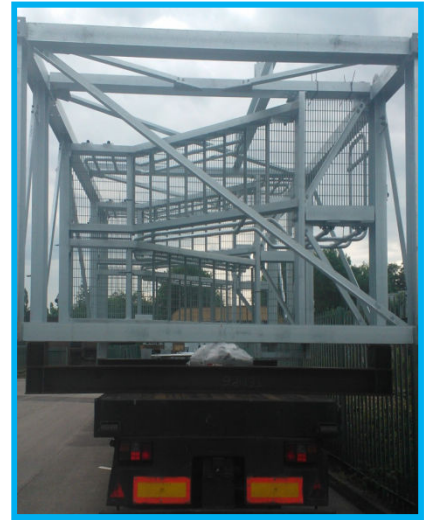
Loaded on the Trailer
