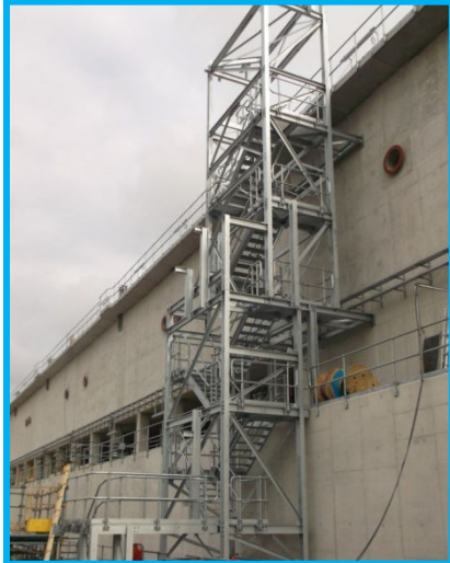
Erected Stair Units
