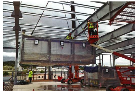
Module delivery and installation
