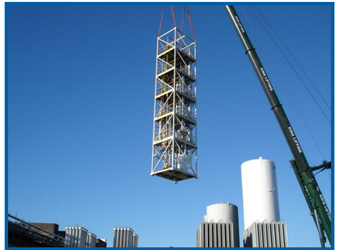
Module Being Erected
