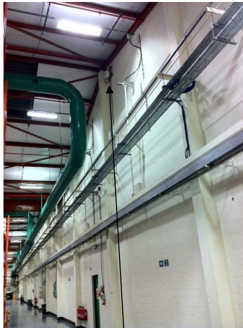
Beam head in situ
