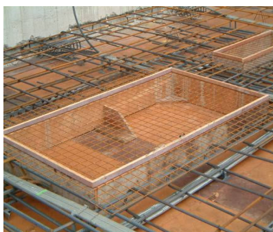
3. Small cast-in metal mesh prevents falls in open areas (though standing on it as pictured may not be advised)
