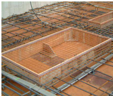
3. Small cast-in metal mesh prevents falls in open areas (though standing on it as pictured may not be advised)
