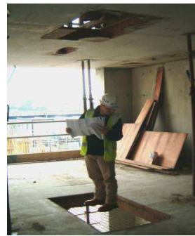
3. Small cast-in metal mesh prevents falls in open areas (though standing on it as pictured may not be advised)
