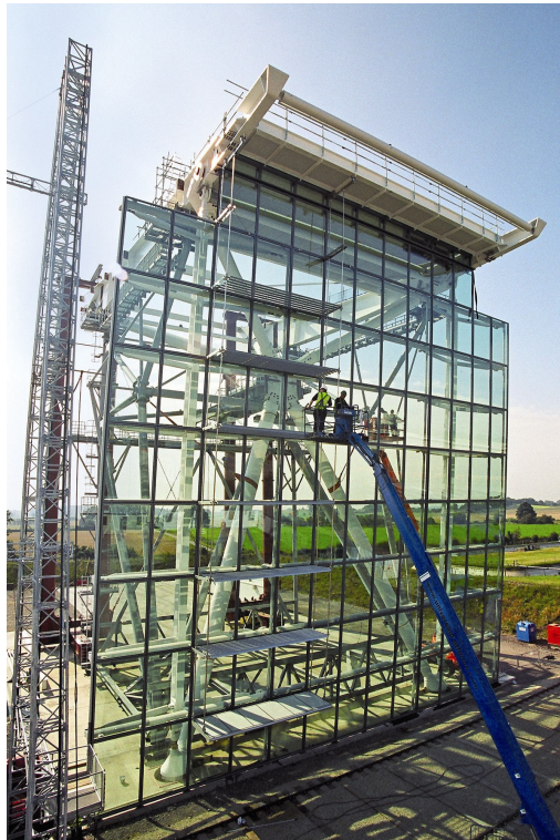
Full size mock-up of steelwork and curtain wall
