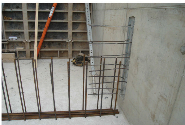
As fitted Eazistrip - vertical joint wall to wall
