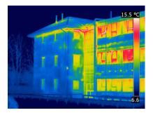
Image shows heat loss from old (right) part of the building with the new building (left) having much better levels of insulation.
