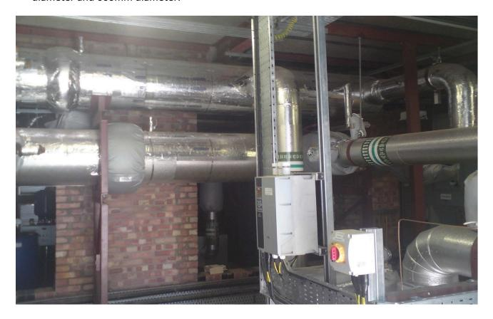
The main benefits of using 3mm thin wall grade 304 stainless steel are the material and labour cost savings, lighter in weight and the speed of installation time, compared to mild steel.
