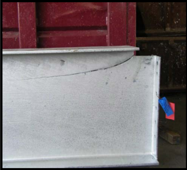
Fig 1 – A Major LMAC Failure
