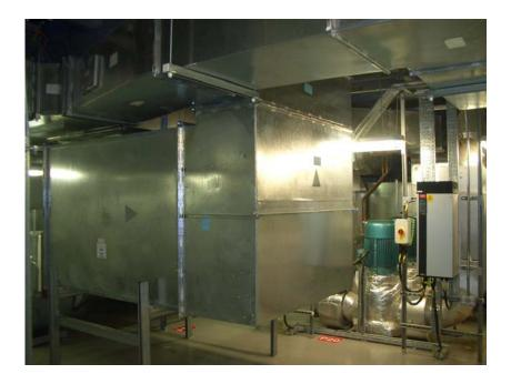
Large bore galvanised fume extract ducts. Achieving the same in PVC ductwork would have considerably higher cost and environmental impact.
