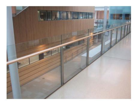
When glass is to be installed at height the main choice is between toughened glass, designed to fail by shattering into small blunt "dice," or laminated glass, which stays as a single sheet when it fails, but requires a sturdier frame to prevent the whole sheet falling out.
