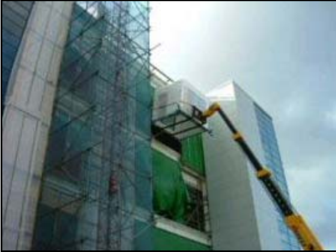
Pod During Installation
