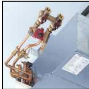
Typical 4port Control Valve arrangement for LTHW/Chilled water to Fan Coil unit utilising Dominator Z3000.
