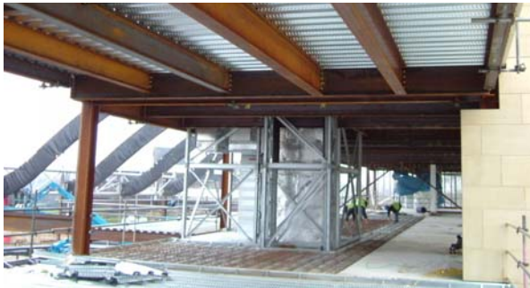
A Typical View at Floor Level
